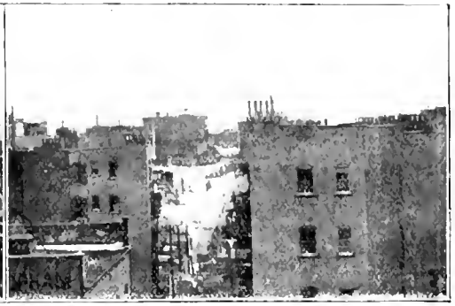
FIG. 10. "WASH OUT ON LINE."
